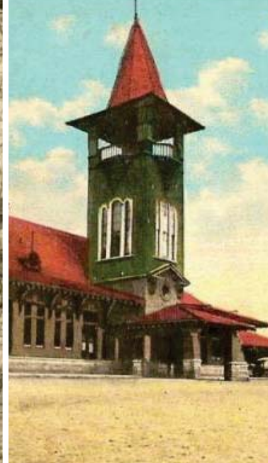
SOUTHERN RAILWAY PASSENGER STATION
