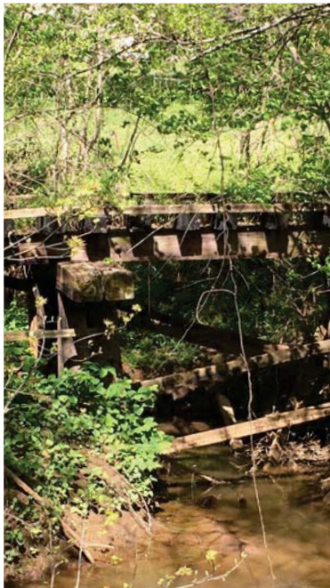
TIMBER RAIL BRIDGE
