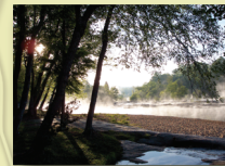
12 Ware Shoals Lake, Dam & Power Plant In the 1920's William Ware built a grist mill near the beautiful shoals, and Benjamin Riegel built a dam and cotton mill at the turn of the century. The mill is gone now, but the town of Ware Shoals is capitalizing on the beauty of the shoals and on the town's rich history to create a master plan for redevelopment.
